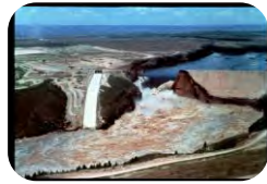
Dam / Levee Failure
