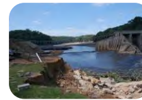
Dam / Levee Failure
